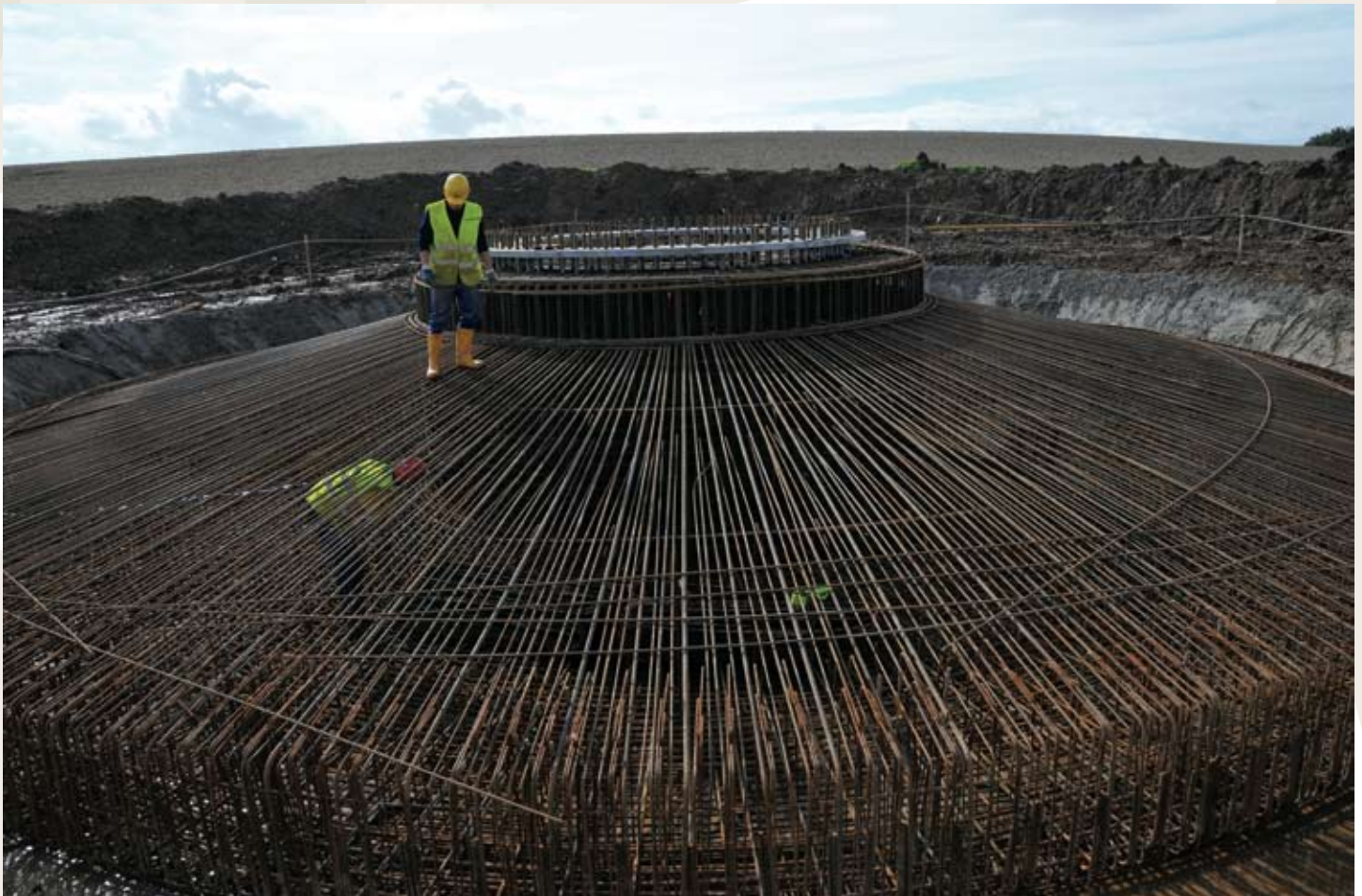
Fig 1. Steel-fixing in turbine foundation
