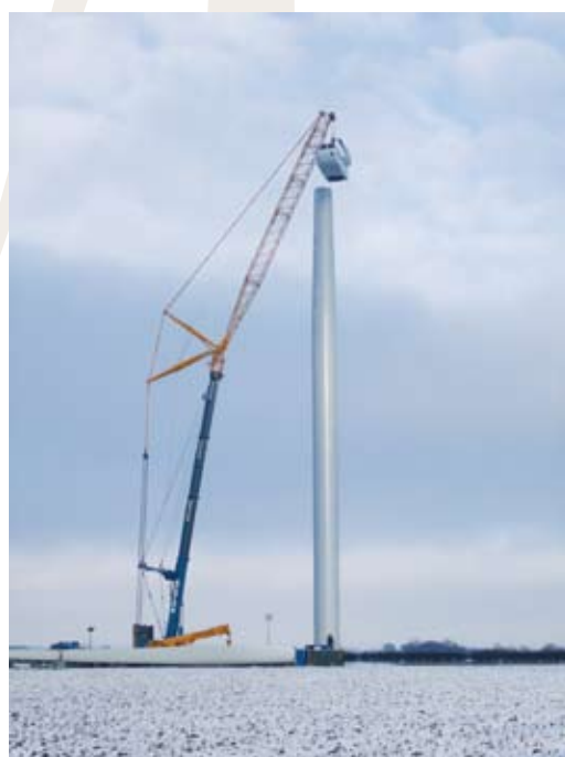
Fig. 2 Turbine erection works
