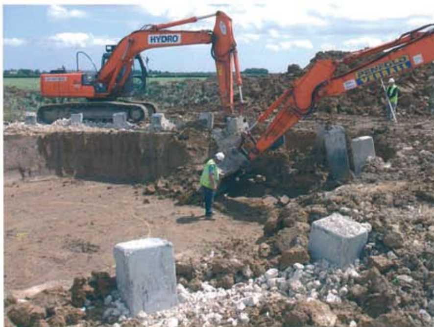
FIG. 2 EXCAVATION OF TURBINE BASE TO FOUNDATION LEVEL
