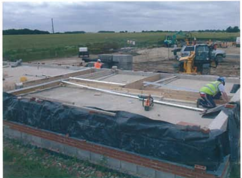
FIG. 1 WORKS AT WIND FARM SUBSTATION
